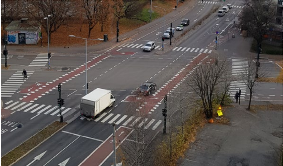
FIGURE 4-37 Solution with wide left turn at intersection in Lovisenberg.
