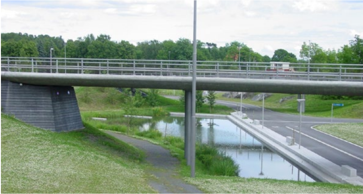
FIGURE 6-3 Example of open dam to retain and clean stormwater from the road.
