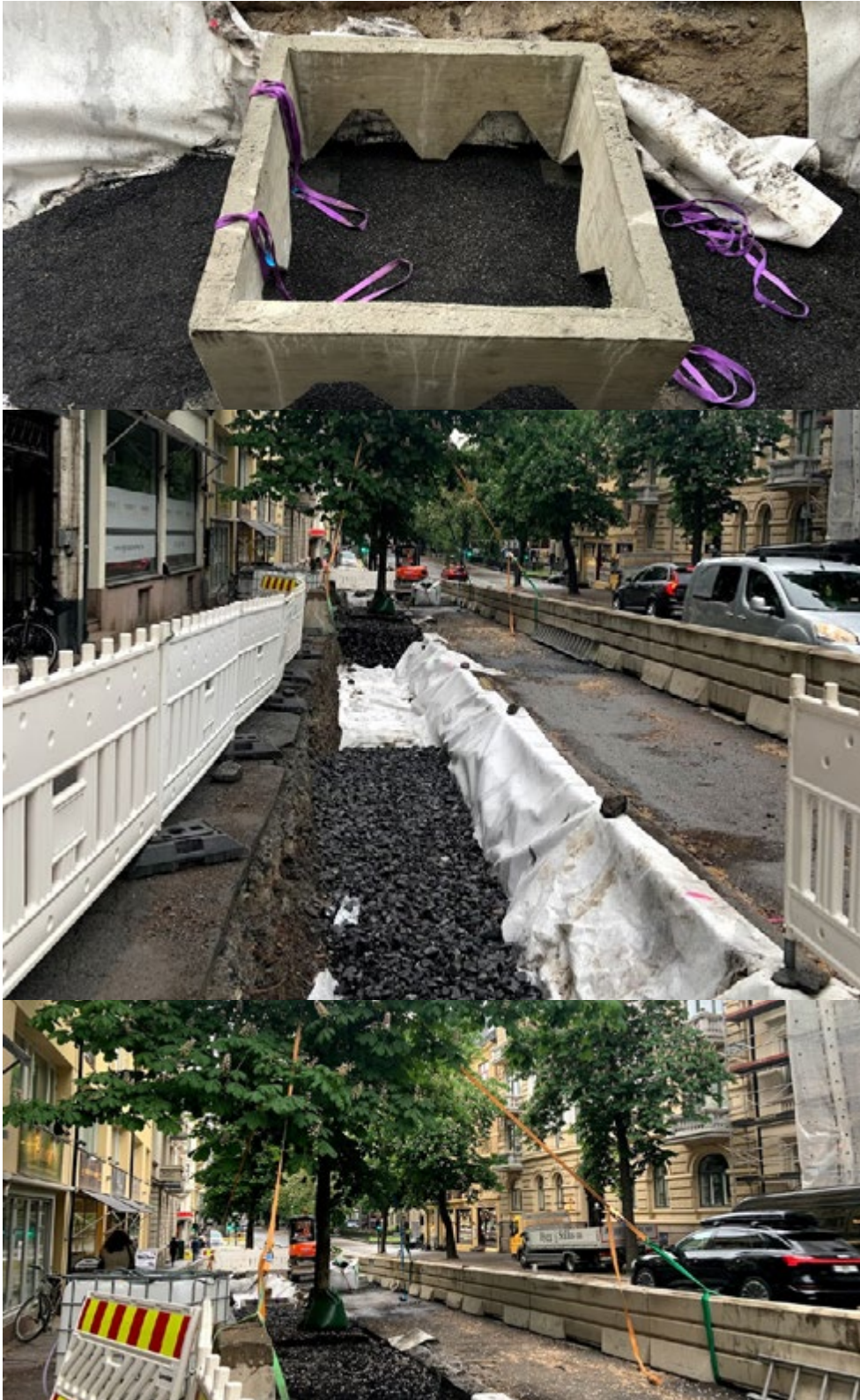
FIGURE 7-17 Example of a root reinforcement layer and biochar laid on Bygdøy Allé.
