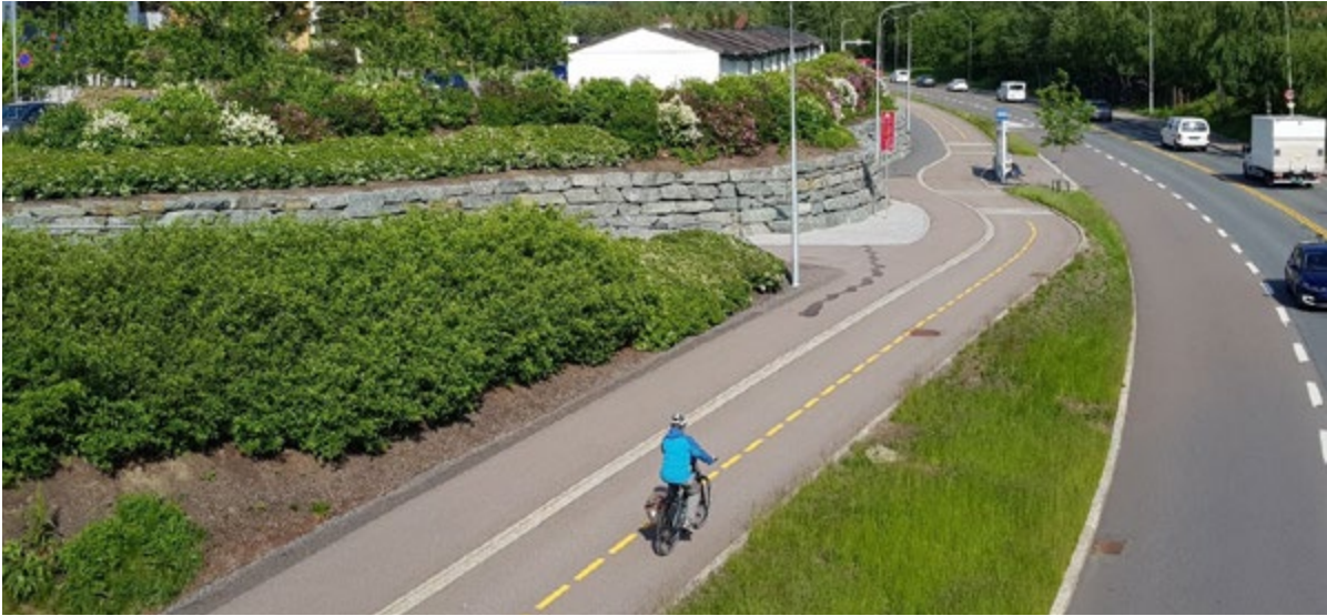
FIGURE 4-13 Cycle path with pavement on Tvetenveien.
