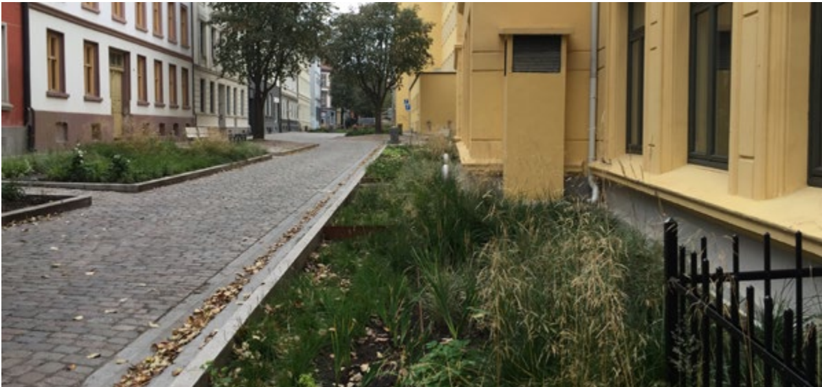
FIGURE 2-8 Deichmansgate is an example of a type B1 street.
